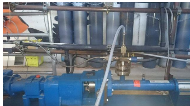
Figure II.3 – Moineau® pump (PCM Instruction Manual).
