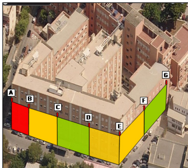
Fig. 4.2; Example of representation of noise on the façades of a building, using colours to indicate different noise levels, as proposed in the second test.
