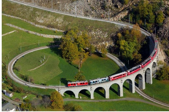
Figure 51 Spiral viaduct near Brusio, Switzerland [bahnbilder.ch]
