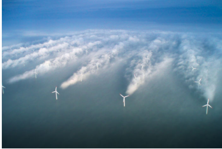
Figure 1.1 – Wake of wind turbines revealed by fog (Hasager et al., 2013) on the offshore wind farm, Horns Rev 1 in the North sea. Turbines within the array can be seen to be operating in the wake of upstream turbines. (80 wind turbines, 160 MW of production capacity.)
