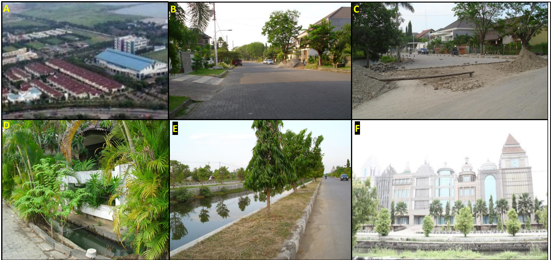
A. Aerial photo of Puri Marina Area B. Paving as primary street C. Street reconstruction D. Inundated local drainages E. local canal (drainage) F. Commercial and Business buildings
