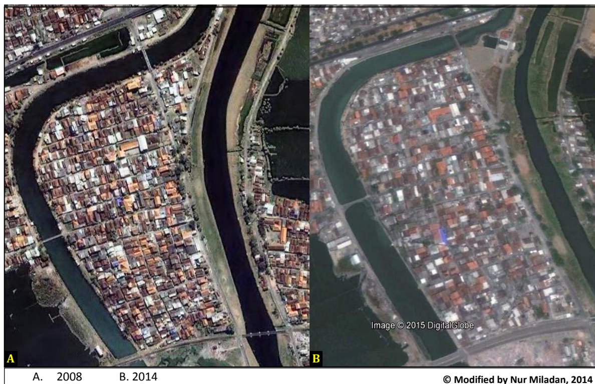
Figure 177. Land use transformation in kampung Cilosari: Pumping house area
