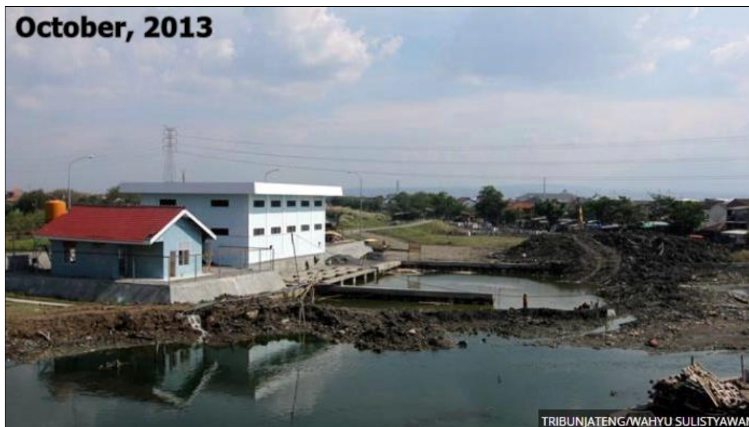
Figure 71. Construction of the pump station area of Banger Polder Project has not been completed
