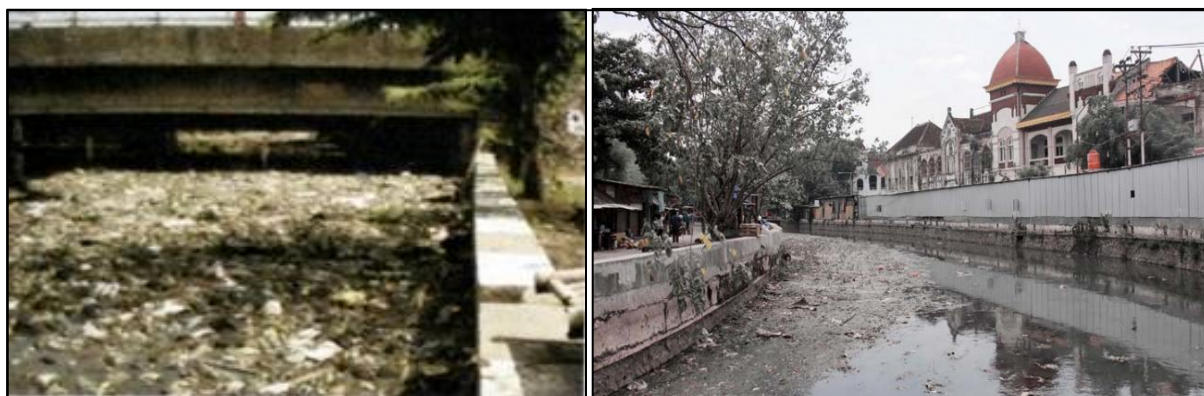
Figure 59. Waste on the urban drainages of Semarang City
