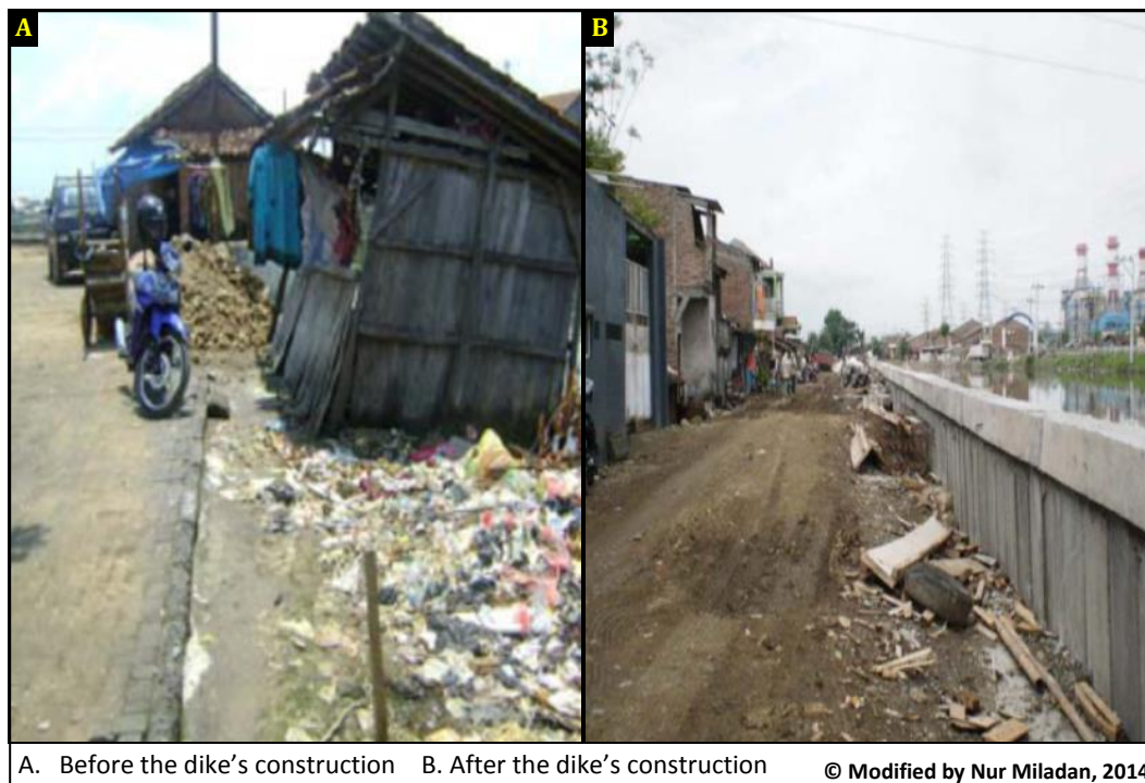
Figure 178. Construction of the north dike around kampung Cilosari in 2010
