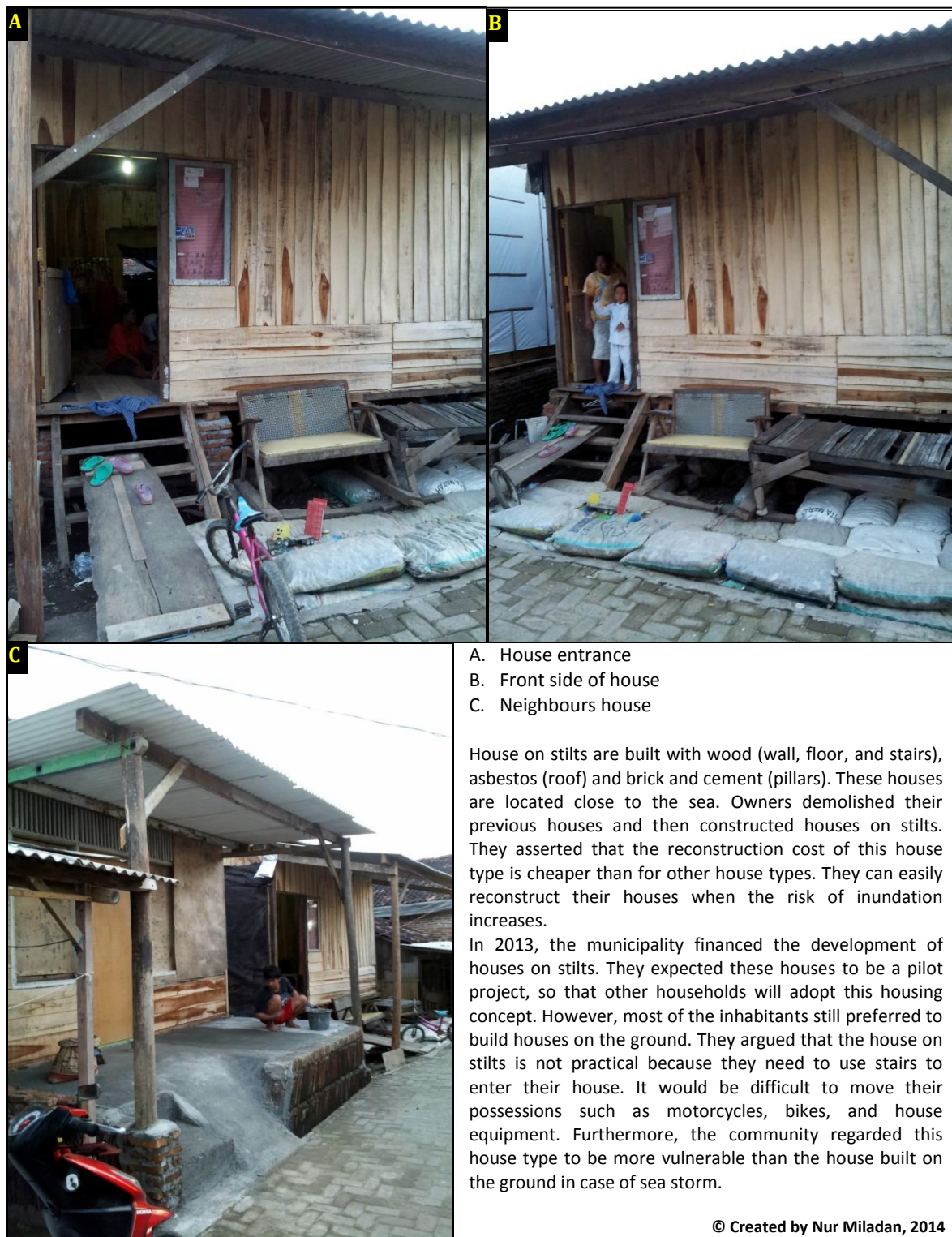
Figure 147. House on stilts in kampung Tambak Lorok
