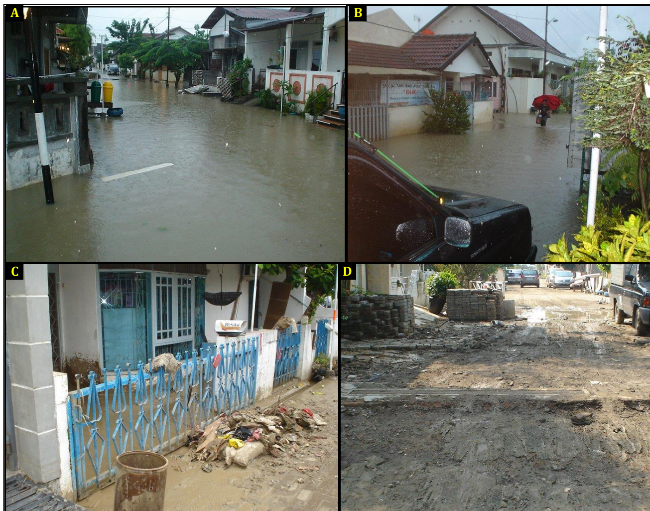
Figure A and Figure B indicate that during the flood occurrence, the inundation level was between 0.5 m and 1 m within the settlement. Meanwhile, Figure C and Figure D describe the settlement situation after the inundation: street destruction, waste and mud dirty everything.
