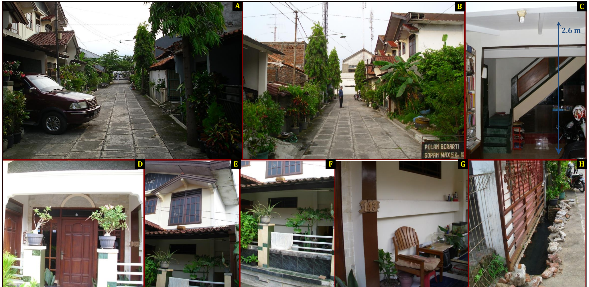
Figure A and B describe the house sample situated near a street (4-5 meters long). The house is higher than the surrounding houses. Figure C indicates the distance between the roof and the floor inside the house is only 2.6 meters. It was initially 4 meters. Figure D and Figure E show the front faces of the first and second floors. Figure F features the fence made of cement and ceramic. Figure G describes the terraced wall in the front face. Figure H represents the inundated drainage around the house.
