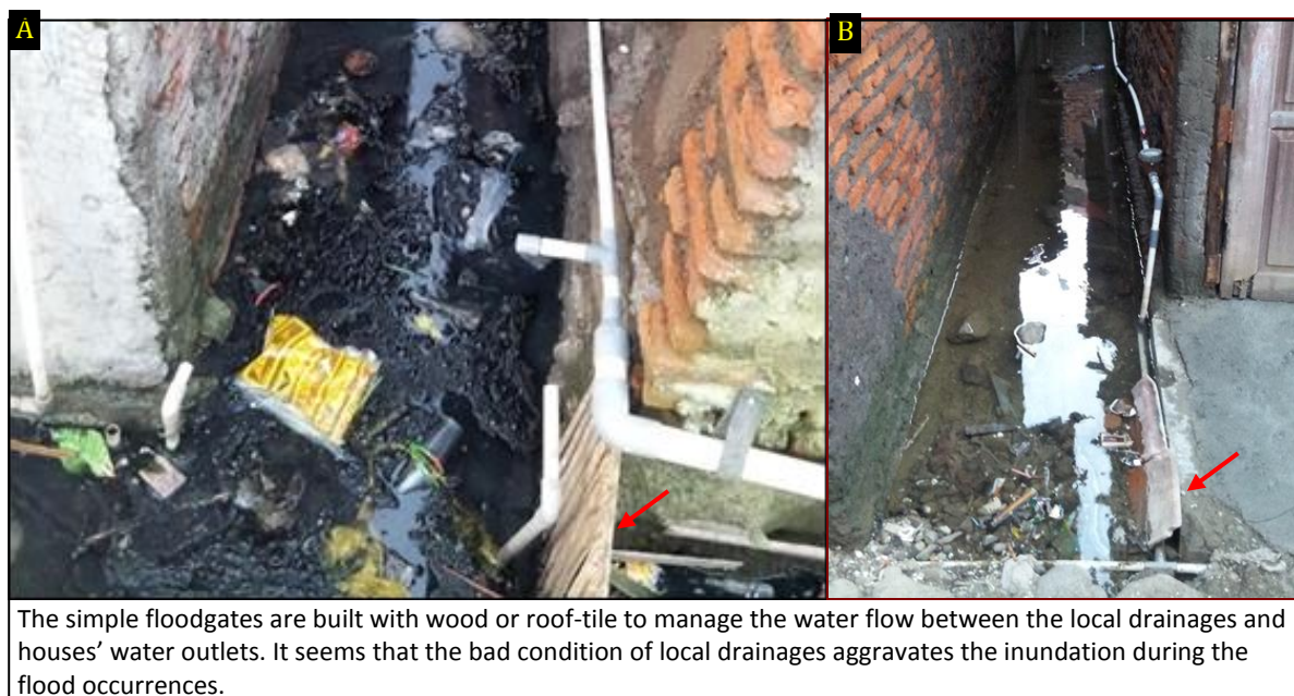
Figure 162. Simple floodgates between local drainages and houses' water outlets
