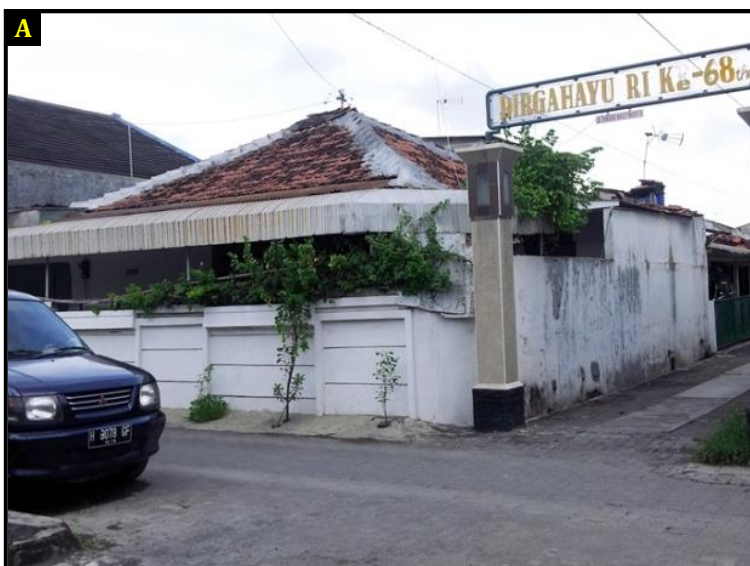
Figure A: A house is surrounded by a solid fence to reduce the inundation risk. However, the house has not a proper air circulation and also the sunshine cannot enter.
