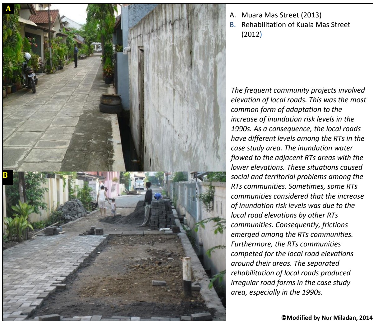
Figure 111. Rehabilitation of local streets in the case study area
