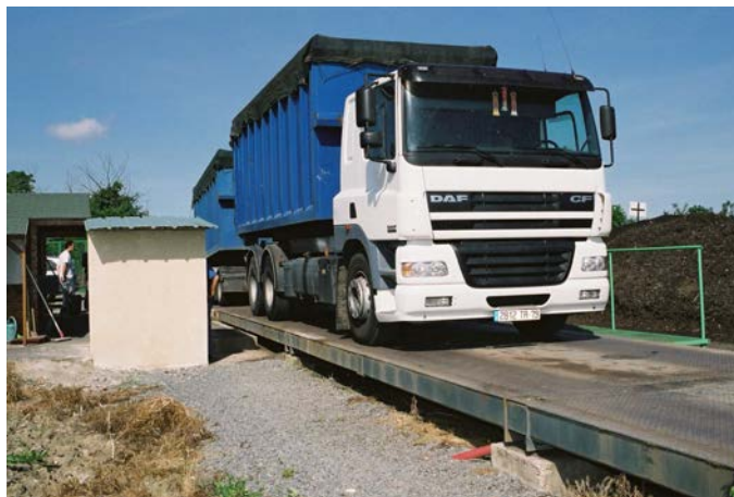
Figure 3.5: Weighbridge in a powerplant.
