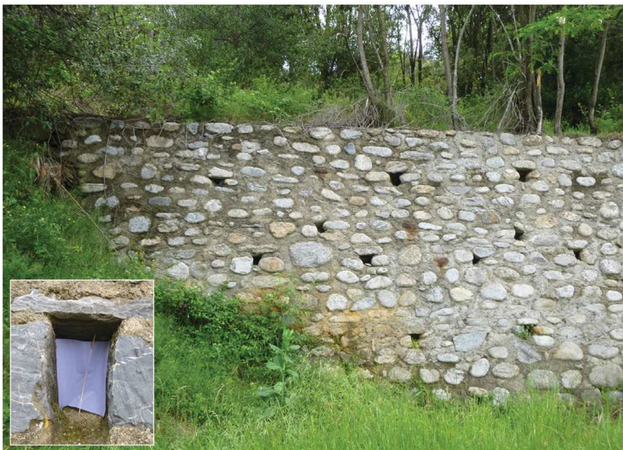
Figure 3. Station No. 3. Trapping wall with weep holes (or so-called “barbacanes” in French). Inset: a weep hole containing a sticky trap. Forefront: Brachypodium phoenicoides meadow along the edge of a road. Background: Robinia pseudacacia and Quercus ilex .
