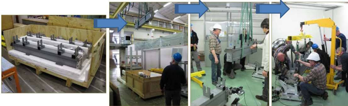
Figure 4-19: Delivery and assembly sequence of the supporting system for Case B
