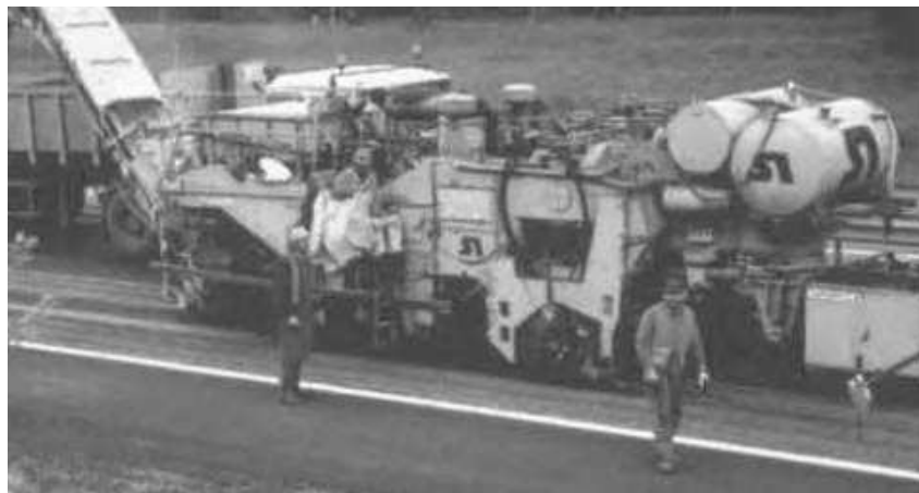
Figure 2-20 Breaking up of old asphalt slabs for use as RAP (bitumen.info, 2009)
