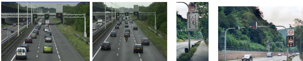
(e) Emergency / Stop lane use and driving orientation reversibility
