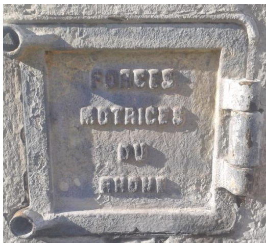
Figure 61 : Coffret mural de raccordement
