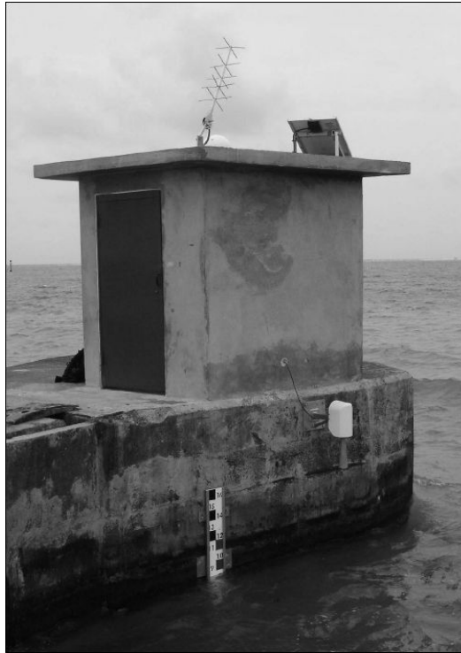
FIGURE 6.4 – The tide gauge station of the Island of Tubuai (inaugurated December 3 rd , 2008.) It is equipped with a GPS permanent station, a pressure and radar sensors (see Fig. (6.3) for precise location.) Tide gauge data (60s averages) are uploaded each 15 minutes to the NOAA GOES satellite (Yagi antenna on top of the structure.)
