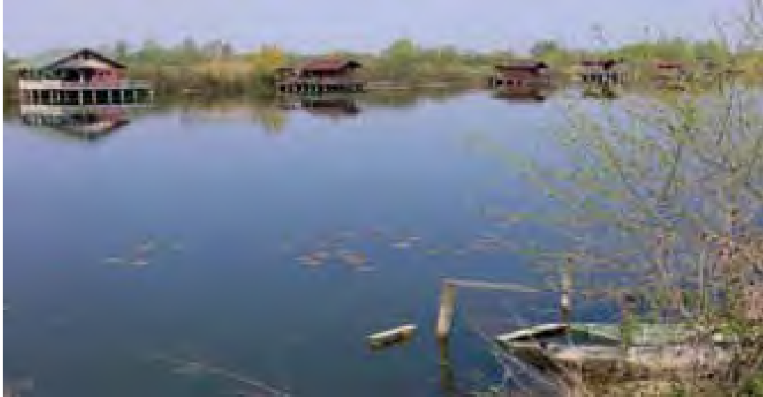
Figure 2.14. An example of how some houses have been built in low laying flood plains. [CNA, 2011].
