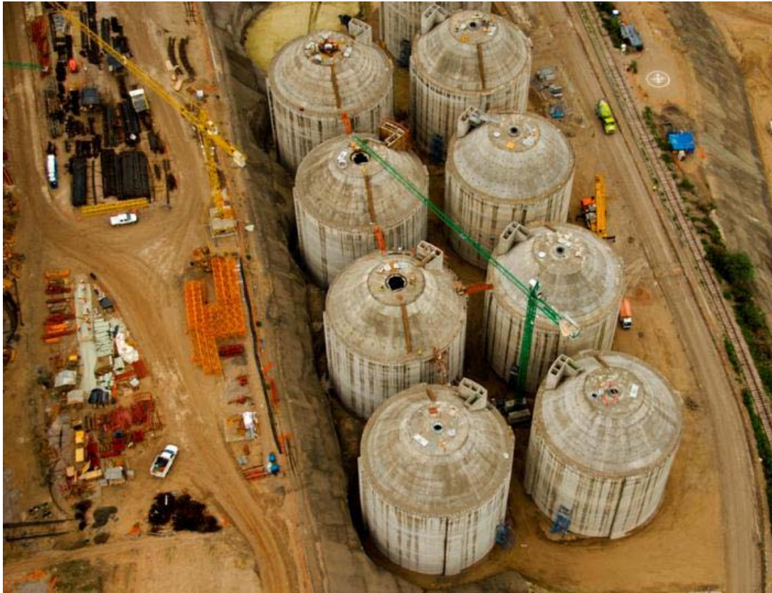
Figure 3.11 Construction of the wastewater treatment plant in Atotonilco. [Luege, 2012]
