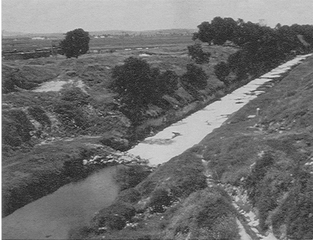
Figure 3.1 A view of the Grand Drainage Canal (Gran Canal Desague), which carries wastewater and stormwater runoff from the Mexico City Metropolitan Area. The canal exits the Basin of Mexico through the Tequisquiatic tunnel and empties into the Moctezuma River, a tributary to the Panuco River, which flows into the Gulf of Mexico. [Luege, 2012]
