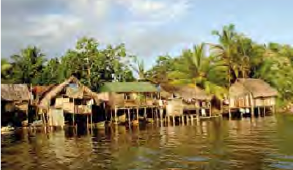
Figure 2.15 An example of how to build houses in flood plains in medium altitude areas. [CNA, 2011].
