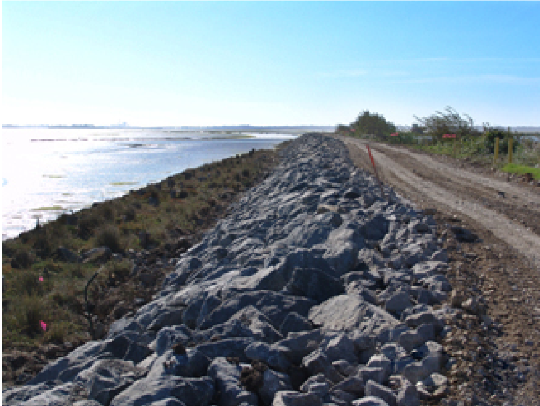
Figure 1.5 Coastal levees protecting Arcata waste water ponds from Humboldt Bay, California. Without levees protecting them, the waste water ponds flooded frequently. [California Gov, 2016]
