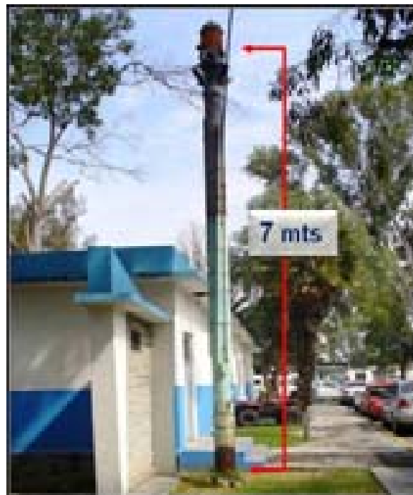
Figure 3.8 Water pump showing the soil subsidence. [Luege, 2012]
