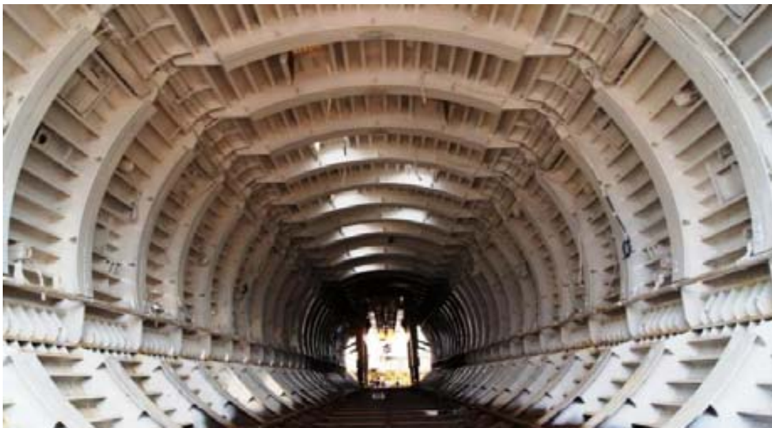
Figure 3.10. East Drain. View of the final lining work with slipform. [Luege, 2012]
