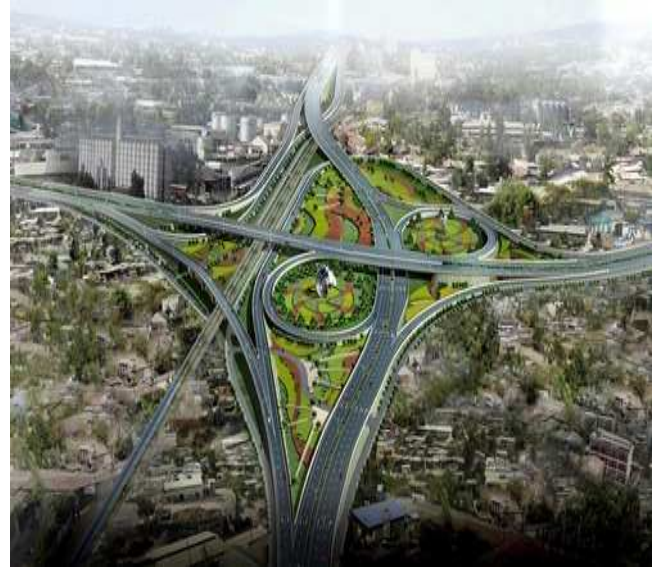
Figure 2.36: The grade separated Gottera Interchange: A major landmark in the city
