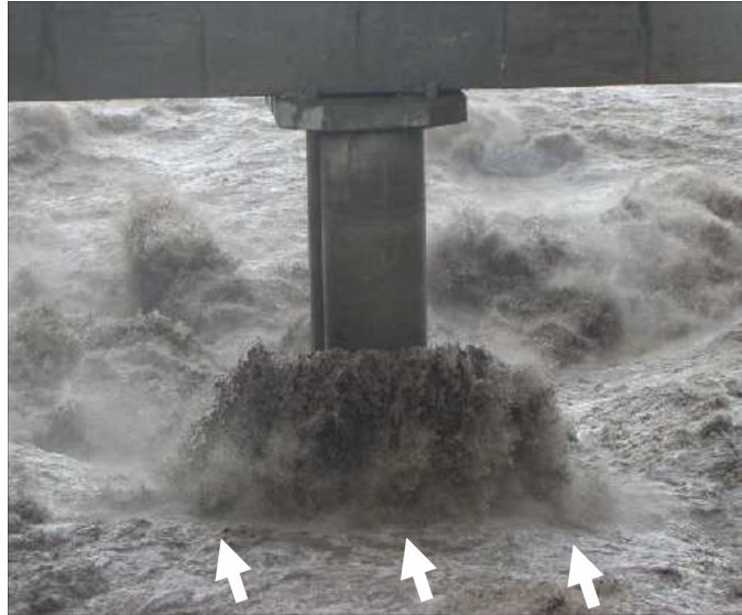
Figure 1. Photograph of the wall-jet-like bow-wave around a bridge pier in the "Rivière des Galets", La Réunion Island, France, in March 2006. Courtesy of Paul Bonnet, DEAL 974 (ex DDE 974)
