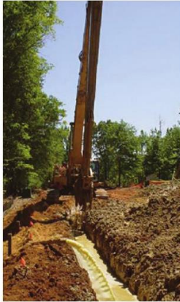
Figure 1-8 Biopolymer trenching (Naidu and Birke, 2015)
