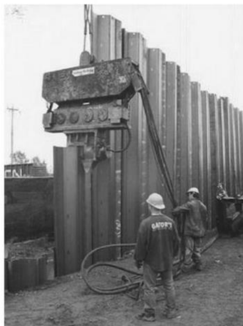
Figure 1-9 Sheet piles installation (Naidu and Birke, 2015)
