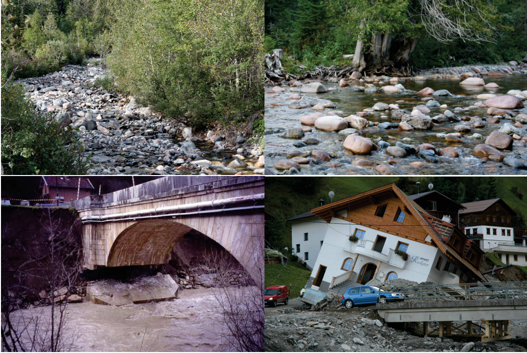
Figure 1.1: Bedload transport: typical streams and related issues. Credits for the pictures: P. Frey, P. Frey, F. Liébault and M. Chiari.
