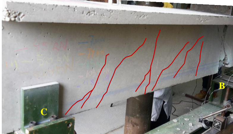
Figure A. 16. Cracking pattern Sample 4.
