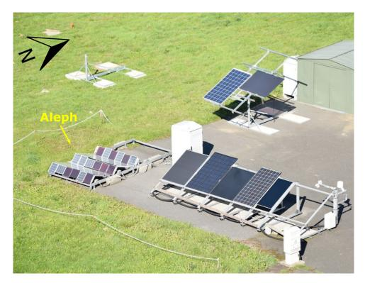
Figure 1-14: Aerial view of the three PV systems installed in SIRTA: Aleph (left center), tracker (right top) and classical fixed-mount (right bottom). Photo credit: Jordi Badosa
