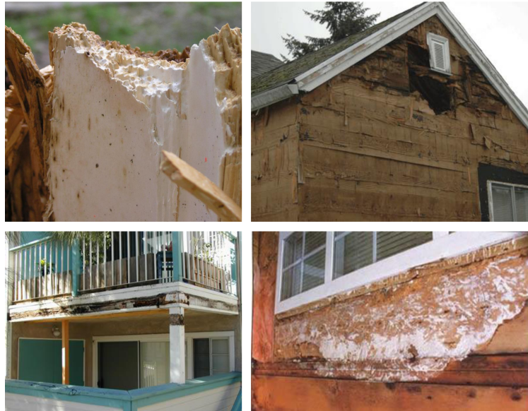
FIGURE 1.1 – Examples of fungal decay on wood in buildings [6, 7].
