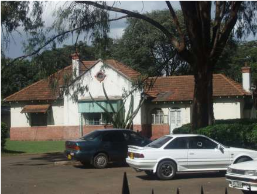
A Railway Officer's house constructed in the early years (1900s) and still standing
