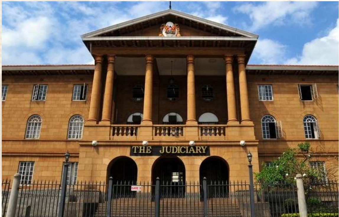
The High Court was built in 1932 to 1934.
