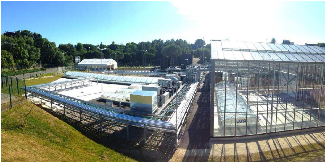
Figure 28 Algosolis platform, Saint-Nazaire, France [111]
