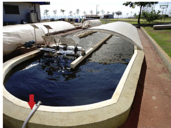
Figure 18 Partially covered raceways for microalgae cultivation at Ourofino Agronegocio, Brazil [48]
