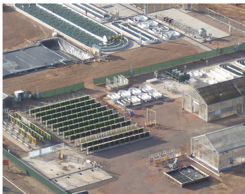
Figure 30 Arizona Center for Algae Technology, Arizona state, USA [113]
