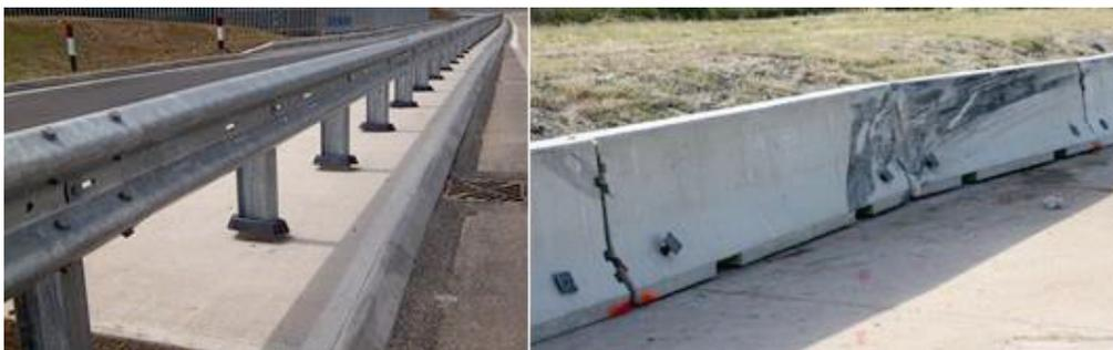
Figure 1- 5 Soft steel permanent VRS and rigid concrete temporary VRS (safety barrier)
