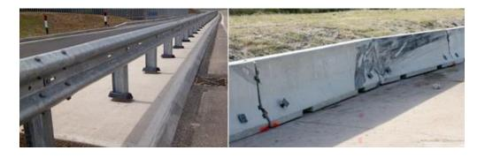
Figure 1- 5 Soft steel permanent VRS and rigid concrete temporary VRS (safety barrier)
