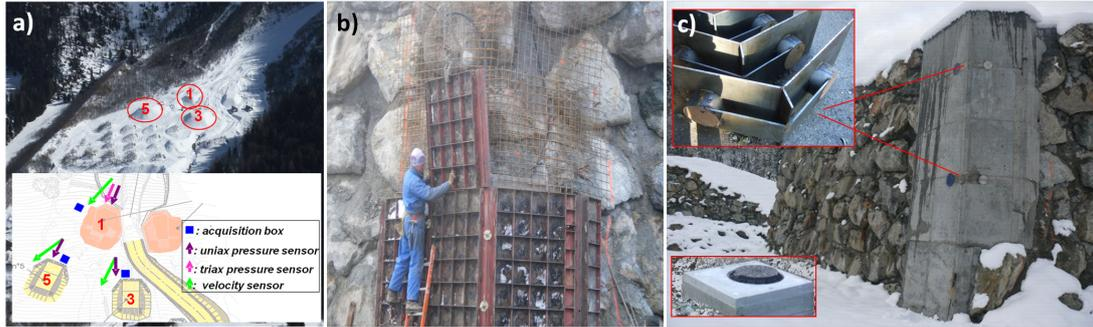
**Figure 3.7:** (a) Site overview and sketch of the three mounds that were equipped. (b) Installation of the reinforced concrete coating on the edge of the mound. (c) View of a breaking mound. The coating support the special pre-cast plates (upper inset) hosting the sensors. The lower inset shows the protective chamber buried at the bottom of each mound where the acquisition units are placed. Photo source Irstea.
