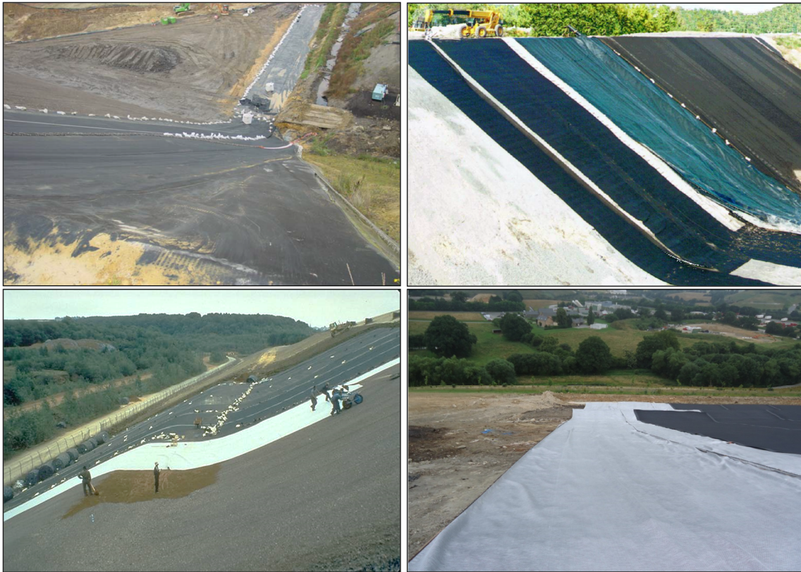
Figure 1.2.2. Landfill covers on slopes.
