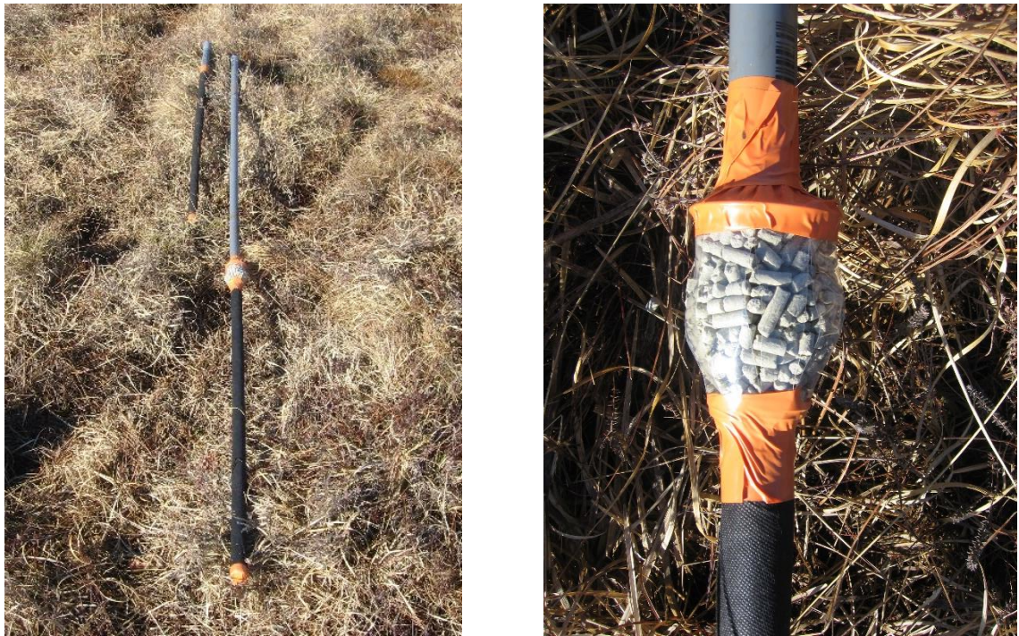
Figure 4-17. Dipwell and piezometer before installation in the ground.
