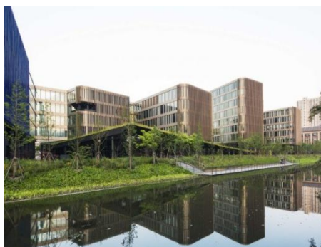
Complexe de bureaux Yidian, Shanghai, 2015
