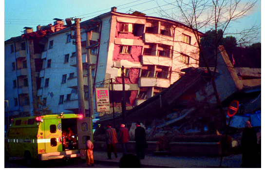
FIG. 1. Tilted building after the Izmit Earthquake, Aug 17th, 1999, Adapazari village, Turkey. Picture: Courtesy of Mustapha Meghraoui, IPGS.
