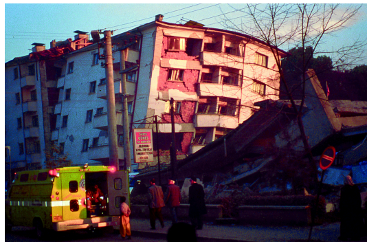
FIG. 1. Tilted building after the Izmit Earthquake, Aug 17th, 1999, Adapazari village, Turkey. Picture: Courtesy of Mustapha Meghraoui, IPGS.
