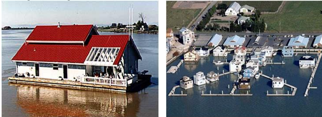
Figure 1.2 Floating homes and hotels
