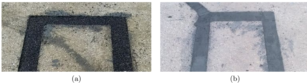
Figure 7.27: Appearance of the hole filled with cold asphalt (a) and MAPEI Mapegrout (b).
