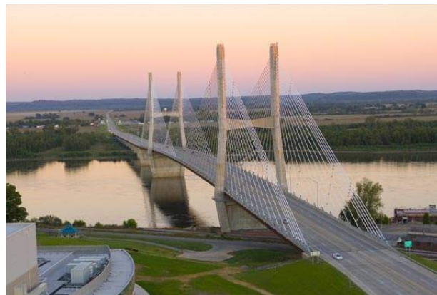
Figure I. 3: Pont Bill Emerson Memorial, Missouri – USA
