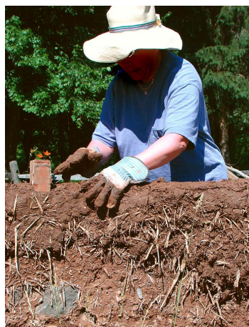
Figure 1.4: Cob wall under construction in France [101].
