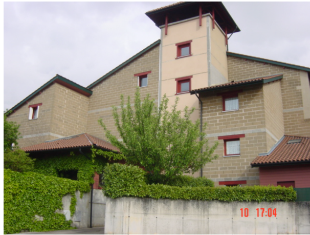
Figure 1.3: House built with CEB (the tower being in rammed earth) in Rhone-Alpes, France [23].
