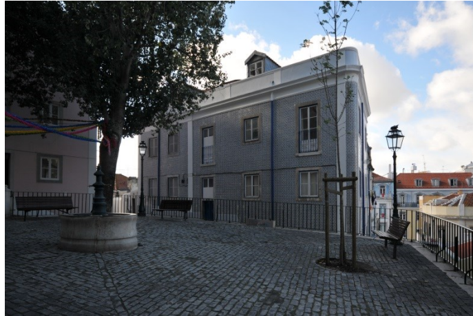
Photographies de Silva Dias Arquitectos
