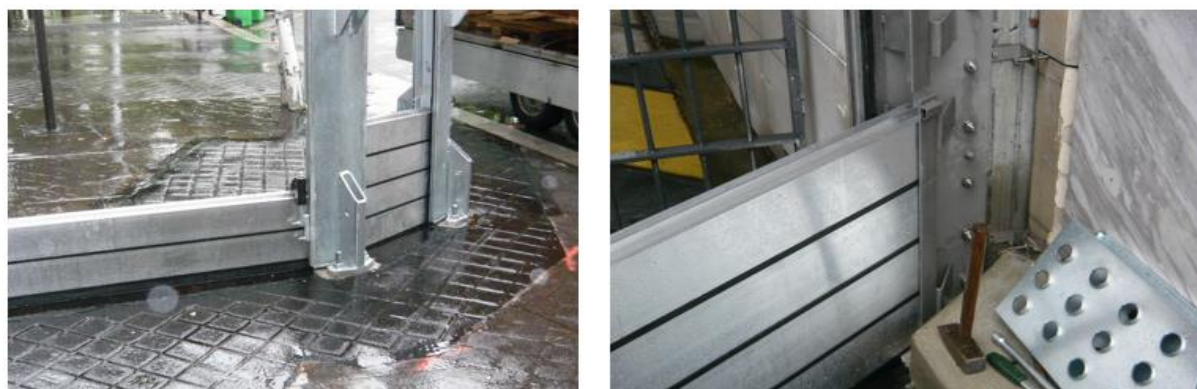
Figure III.E.8. Protections types batardeaux.
