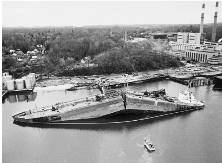
FIGURE 1.1 – Liberty Ship fissuré
