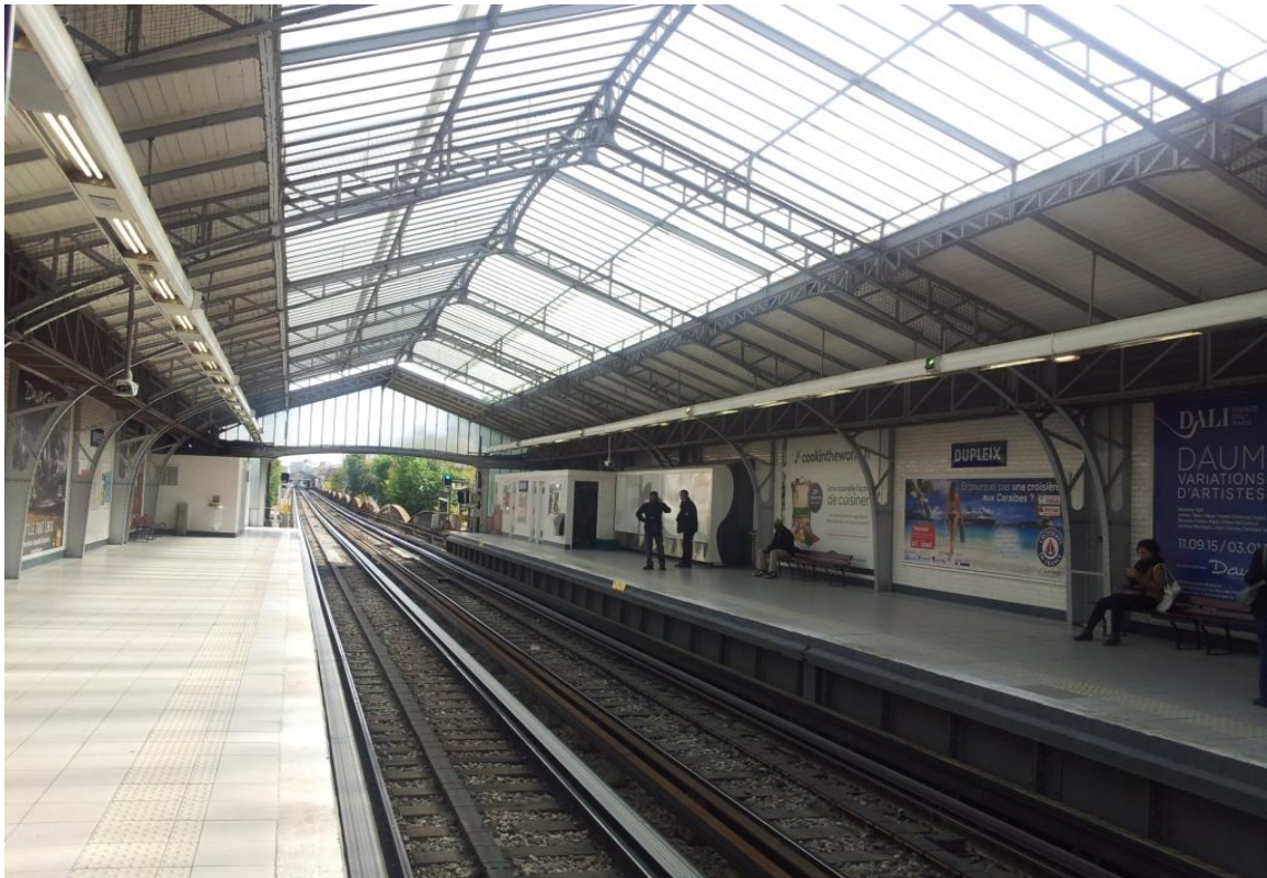
Figure 3 : station Duplex (Paris)
