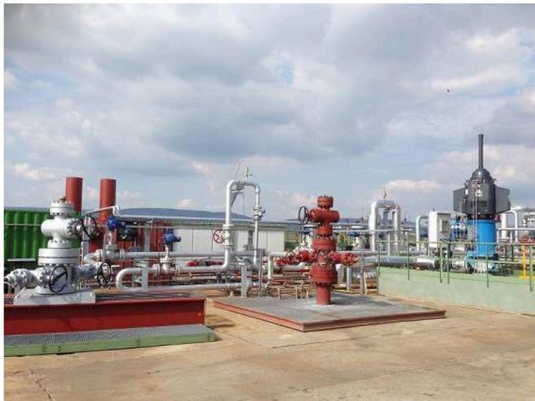
Figure A.1. Surface equipment of the EGS in Soultz-sous-Forêts (wellheads)
