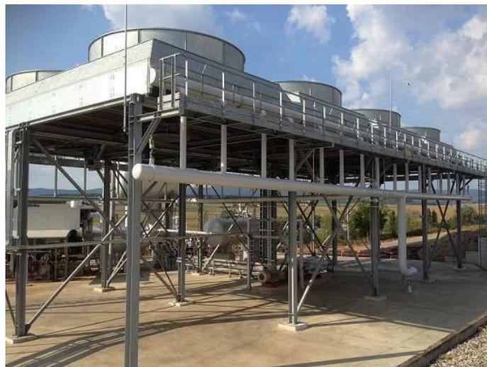
Figure A.4 Surface equipment of the EGS in Soultz-sous-Forêts (aircooler)
