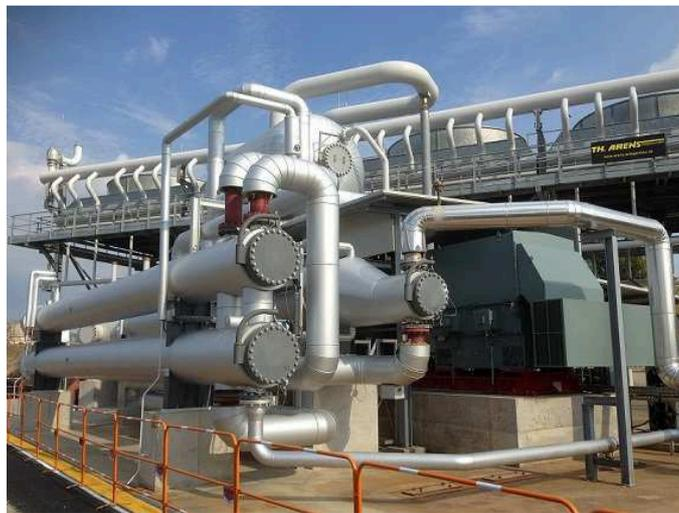
Figure A. 3 Surface equipment of the EGS in Soultz-sous-Forêts (ORC equipment)
