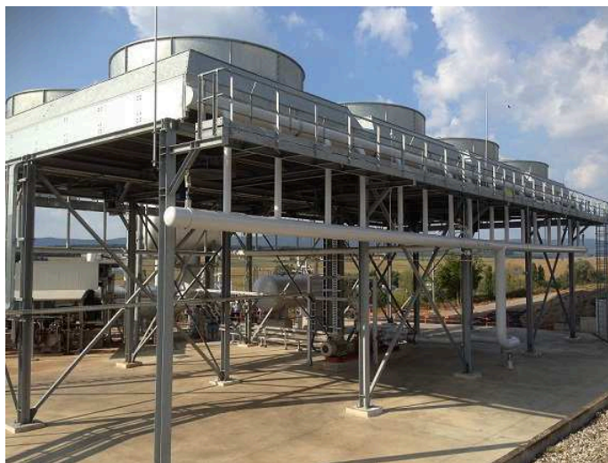
Figure A.4 Surface equipment of the EGS in Soultz-sous-Forêts (aircooler)
