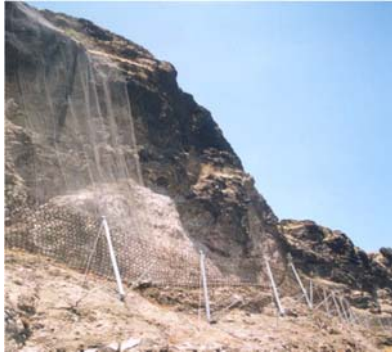
Figure 8 Grillage/filet pendu (CEMAGREF, 2004)
