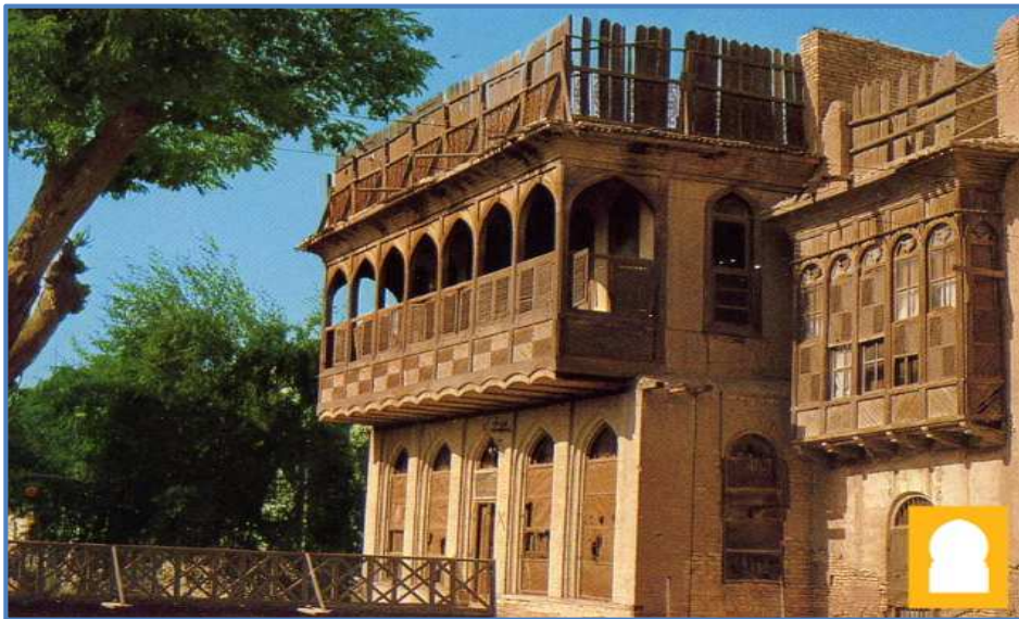
Figure (5-14): View of mashrabiyya in traditional house in Baghdad ( www.google.com ).
