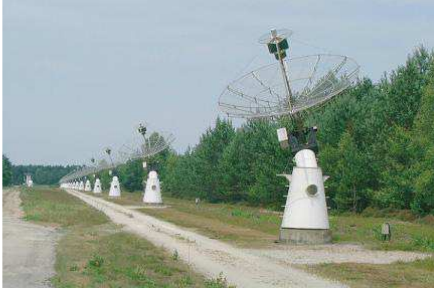
FIGURE 2.2: North-south antenna array of the Nancay Radioheliograph .
