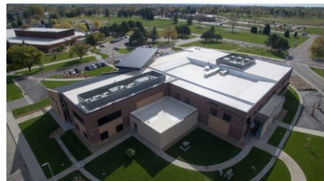
Flat roof (b)
