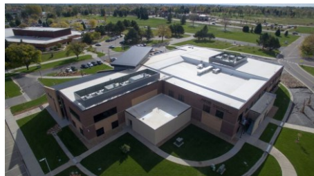
Flat roof (b)
