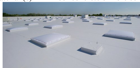
Roof membrane material (f)
