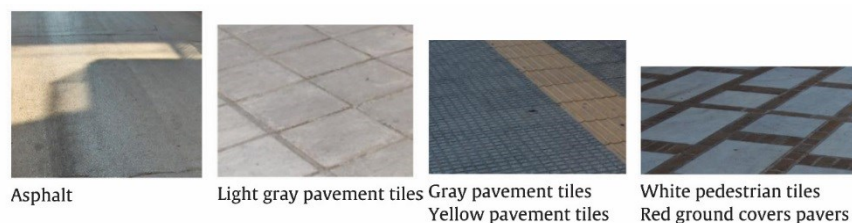
Figure 3. 37: Typical and cool paved surfaces
