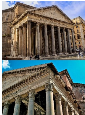
Structural and decorative element
