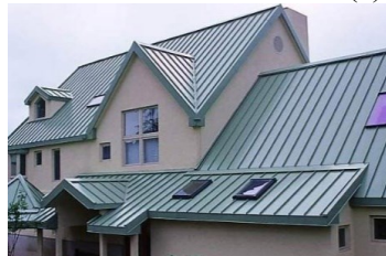
Roof metal material (c)
