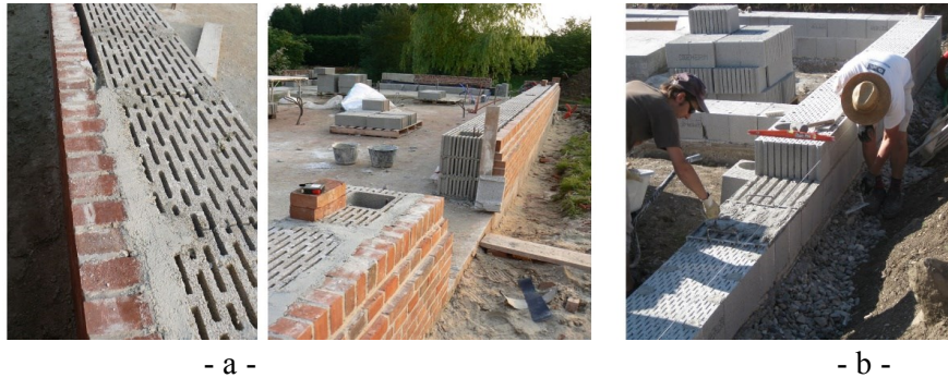
Figure 3. 25: a.Cavity wall insulation, b.Solid wall insulation
