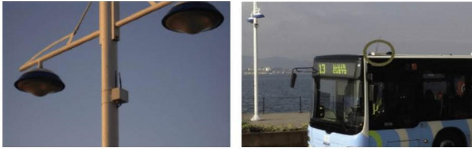
Figure 1.11: Examples of SmartSantander nodes on a lamp post and on top of a bus in the city of Santander [9].
