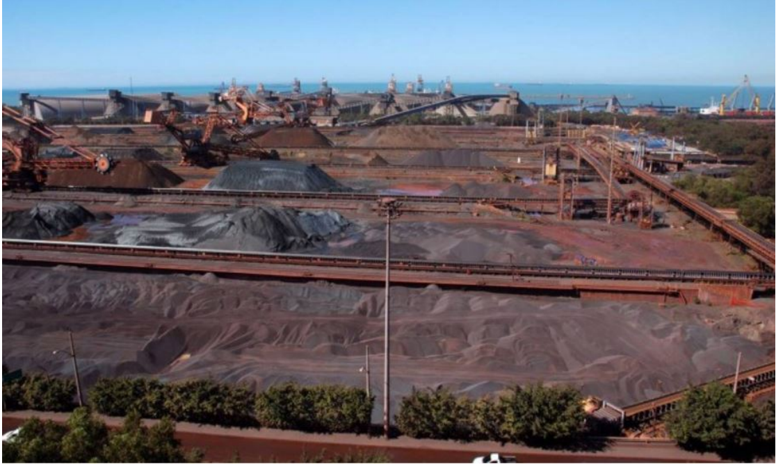
Figure 1: Storage yard of granular material from Arcelor Mittal Tubarão facility, located in Espírito Santo, Brazil
