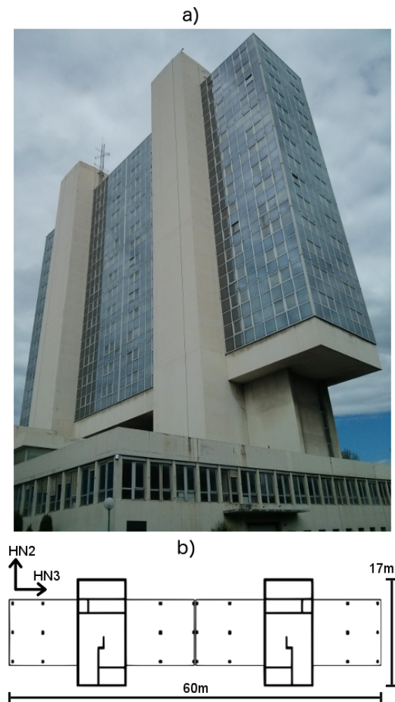
Figure 6.2 – (a) Perspective view of the Nice prefecture building. (b) Horizontal section of building structure.
